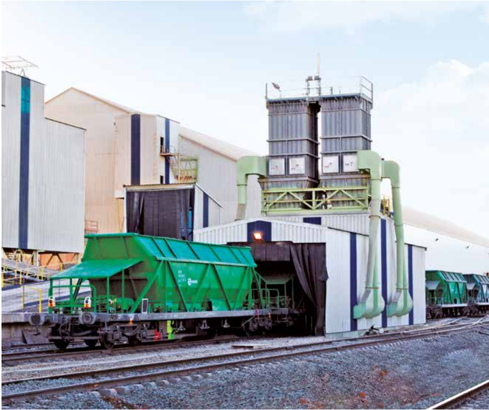
Discharge facility for hopper bottom railcars receives coal for a cement plant including a Samson® Material Feeder with 80 tons holding capacity
