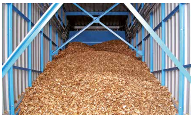
Wood chip intake for a brewery steam boiler
