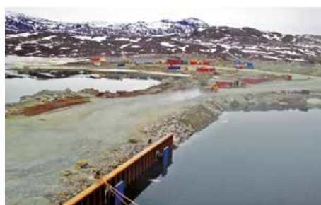
Simple jetty formed in loose rock backfilled
