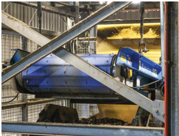
Figure 1 - ElectroMax Overband Magnet in situ on site
