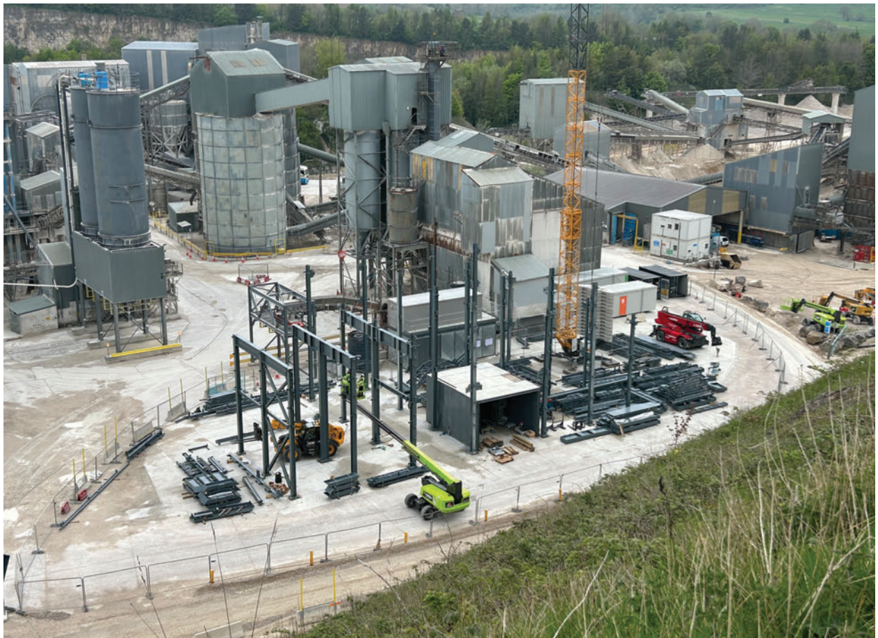
An aerial view shows the progress of the granulation plant construction.
